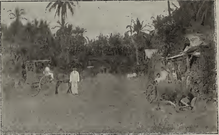
PHILIPPINE HIGHWAY, TYPICAL OF THOSE NOW BEING CONSTRUCTED ALL OVER THE ISLANDS. TWO YEARS AGO LAGUNA MISSIONARIES TRAVELLED THIS ROAD BEFORE IT WAS MACADAMIZED, WITH WATER ALMOST UP TO BED OF VEHICLE
